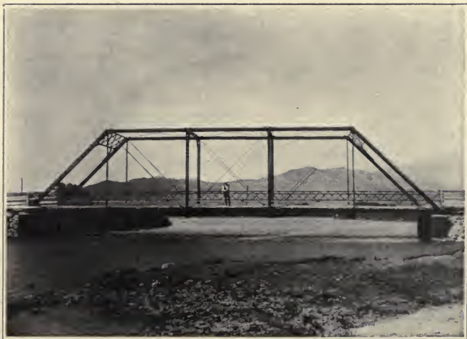
PRESENT BRIDGE ON SITE OF OLD JORDAN BRIDGE.
